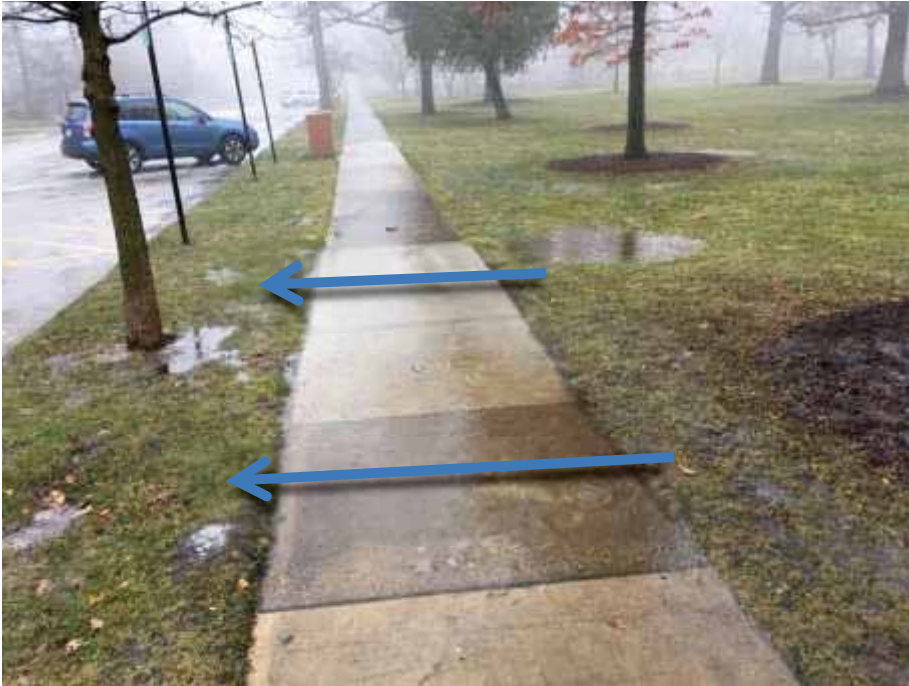
Water Flows Across Paths and Mostly Passes Catch Basin in Park: Need a Delicate Regrade
