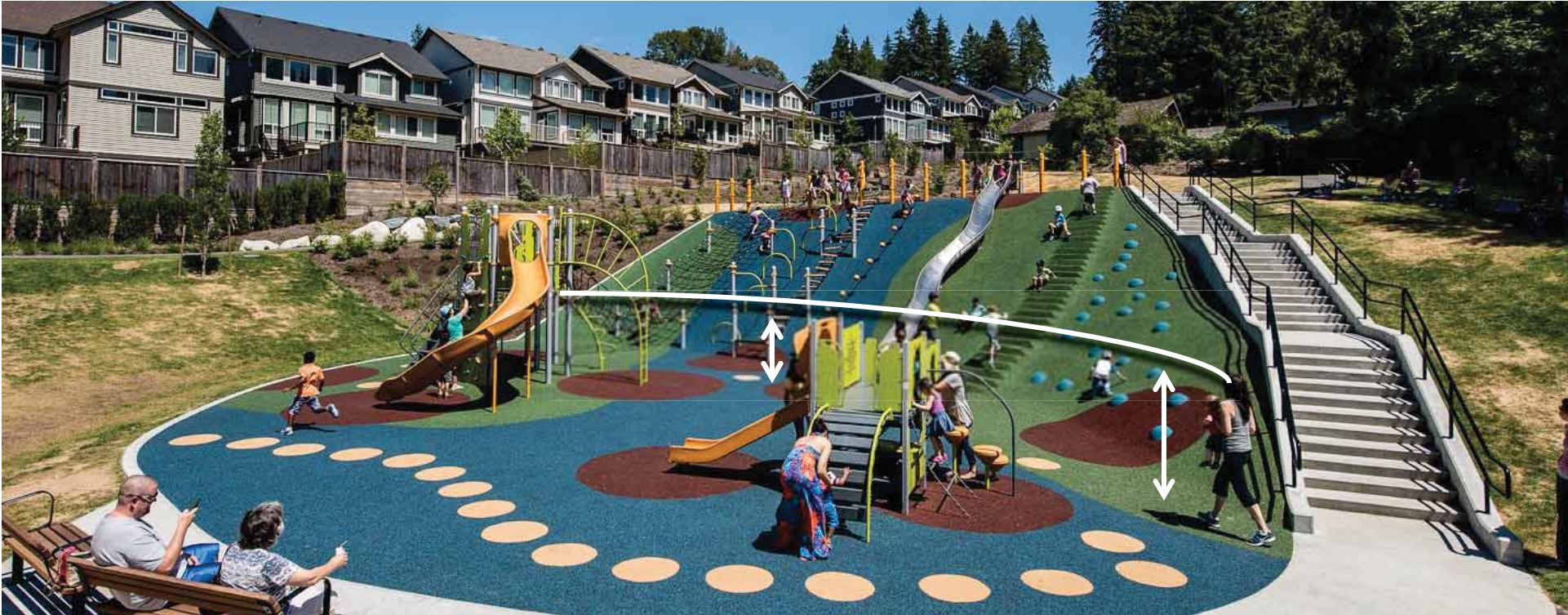
Total existing slope is 5.5 feet over entire playground
