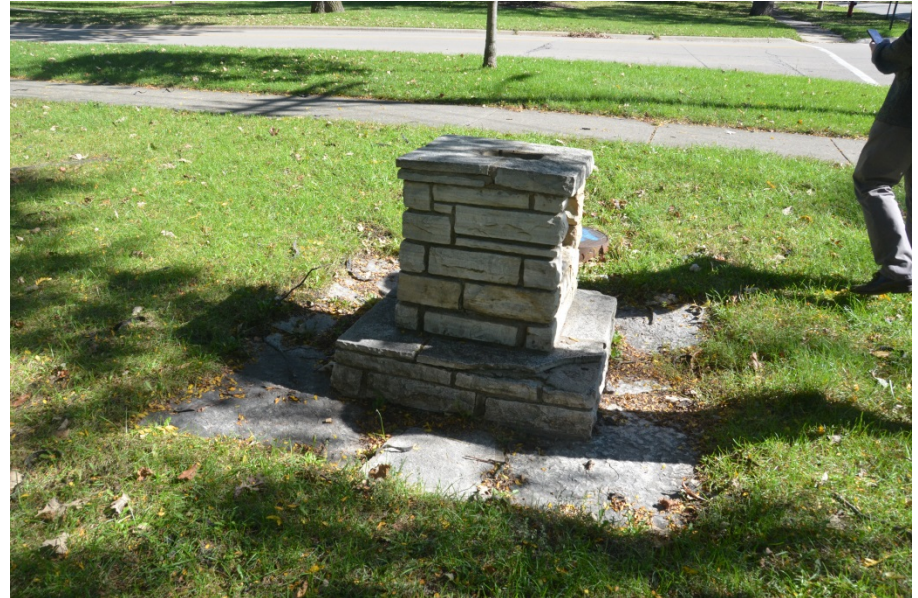
Drinking Fountain at SE Corner of Site
